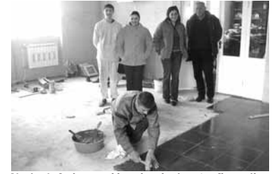
Narine's father and brother laying 1st floor tiles
